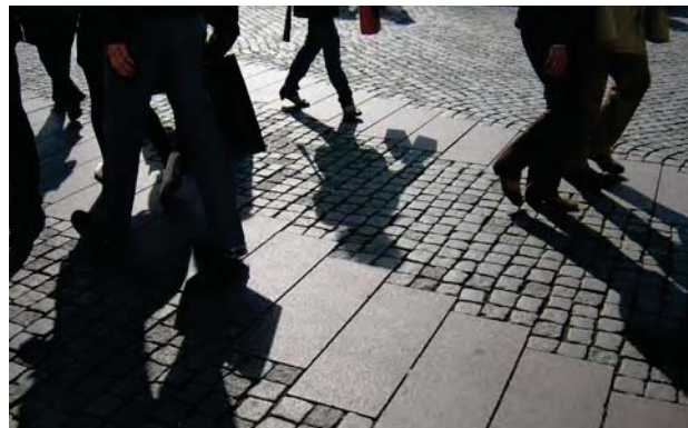
The crossing zone is a mix of different types of pavers, but all of the same material and colour. Malmö, Sweden
