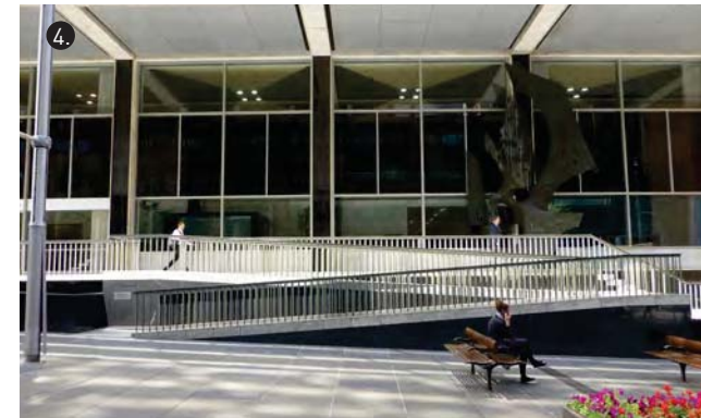
4 Problematic interface between building and square. Reserve Bank of Australia
